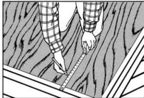
1. Remove all roofing materials for re-roof applications. Install edge flashing & gutter straps as necessary. Measure 5" from edge flashing bend to mark lower slot line. Measure 3/4" further up to mark upper slot line.
