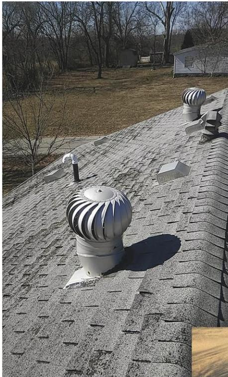
➤ **ABOVE:** Storm-damaged roofs are the perfect opportunity to fix attic ventilation mistakes such as mixing two types of exhaust vents (box and wind turbines) on the same roof. Photo courtesy of Bill West Roofing. **RIGHT:** Box vents have limitations and some roofing contractors in storm-prone markets are getting upgrades covered by homeowners' insurance. Photo courtesy of ABM Services and Renovations.
