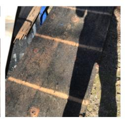
During the callback investigation, Pond Roofing found the insulation packed against the plywood near eaves inside the attic and multiple signs of excessive moisture.)
