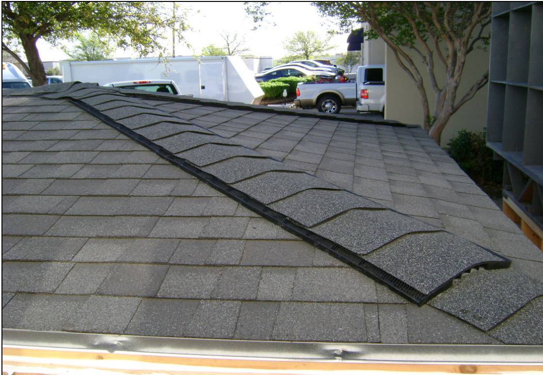
Photo No. 1: Specimen #1 - Wind stream 45° to vent prior to testing
