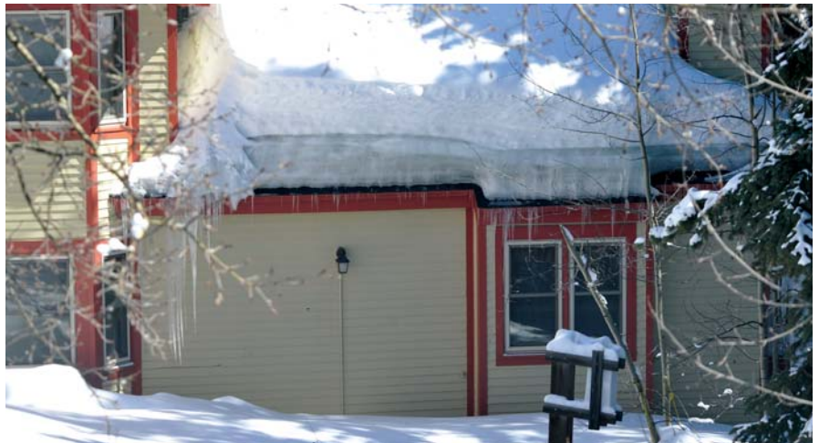
Ice dams of this size weigh more than what the roof is designed to hold. Plus, the water from snow melt seeks the path of least resistance, leading to leaks, mold, and other damage. Photo courtesy of HotEdge.
