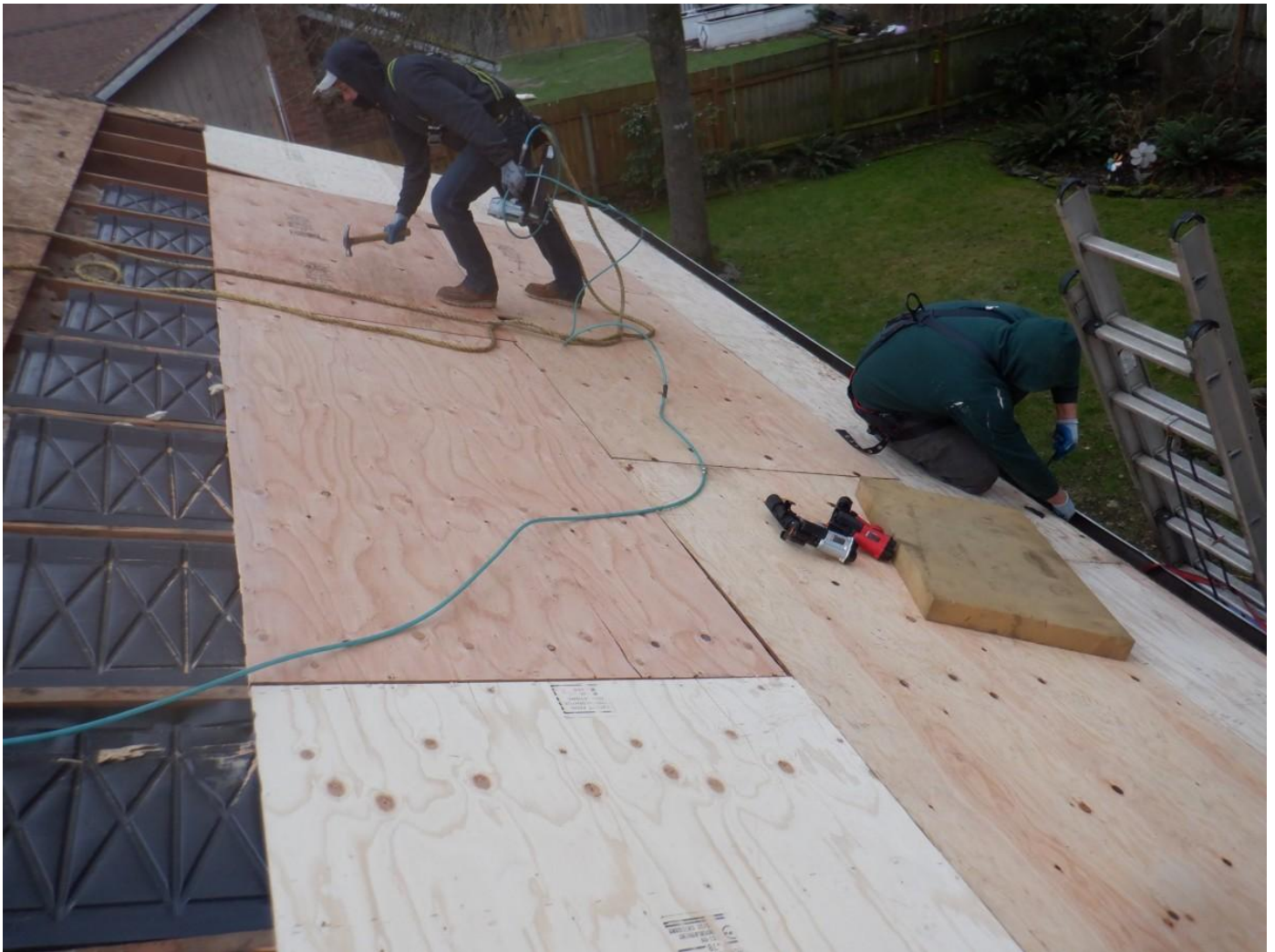
Photos courtesy of Keith Green Construction.
