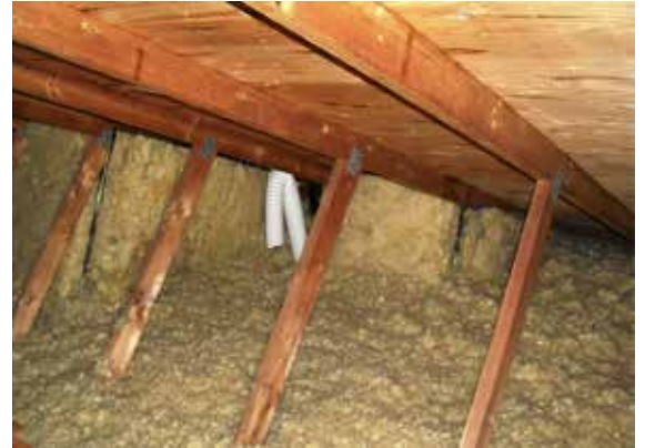
Common ventilation mistakes include bathroom fan ductwork terminating in the attic. Photos: Barry Sigler
