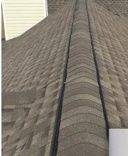
> LEFT: The ideal time to upgrade from box vents that provide localized airflow to ridge vents that allow continuous airflow is during a roof replacement. Photo courtesy of ABM Services and Renovations. BELOW: New exhaust vents installed on the roof need intake vents to perform correctly – unlike this one. Check the condition of the intake vents and confirm nothing inside the attic is blocking the airflow. Photo courtesy of EPIC Exteriors.
