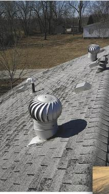
> ABOVE: Storm-damaged roofs are the perfect opportunity to fix attic ventilation mistakes such as mixing two types of exhaust vents (box and wind turbines) on the same roof. Photo courtesy of Bill West Roofing. RIGHT: Box vents have limitations and some roofing contractors in storm-prone markets are getting upgrades covered by homeowners' insurance. Photo courtesy of ABM Services and Renovations.
