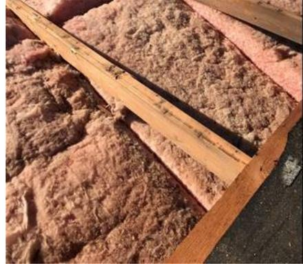
Called back to the house by the homeowner, Pond Roofing Company discovered the insulation packed against the plywood near the eaves inside the attic and multiple signs of excessive moisture. Soon after, Pond Roofing Company would be replacing the roof out of pocket. Photos courtesy of Pond Roofing Company, Fairfax, VA.
